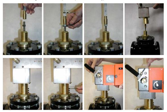
Return pressure to valve, return power and signal to actuator, check operation, and look for leaks. If packing leak is present replace the packing, this time being sure the valve stem is clean and free of longitudinal scratches.
