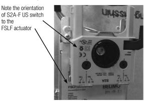
**4A** Note position of hollow shaft adapter for use on FSLF actuator.
