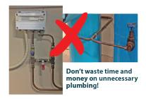
Remote sensors eliminate need for bypasses
