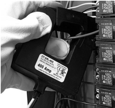
Figure 2. Install CT around Conductor.
